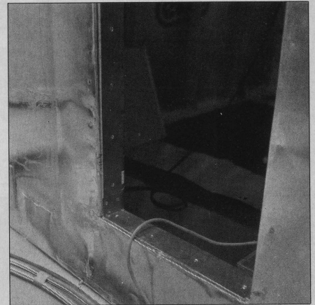
Figure 5. Photograph of personnel doorway close up.
